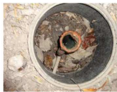
Chem-Rod grounding electrode installed in service well
