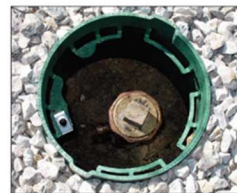
Chem-Rod grounding electrode installed in service well
